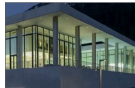
Hallenbad Ovaverva - St. Moritz
