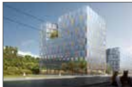
Green City Baufeld C10 - Zürich
